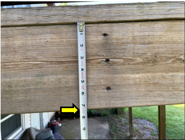
Photo 3 – All support structure 2x8 lumber
